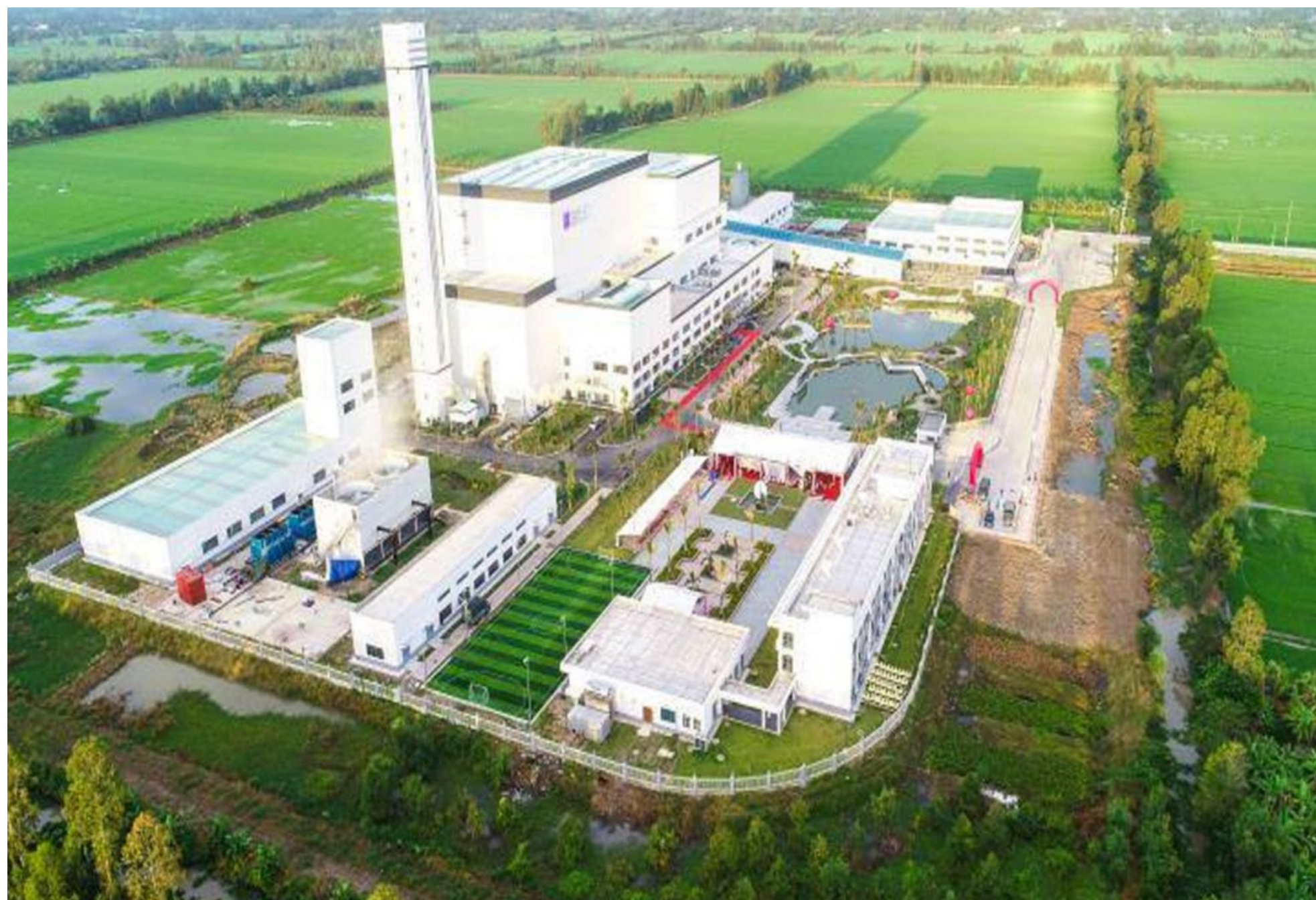
Can Tho waste-to-power plant
